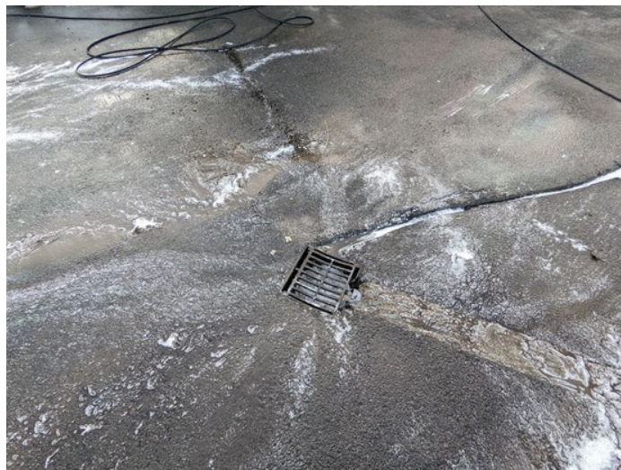
Figure 12: Image from a site highlighting water flow from HCW site. Suffolk
