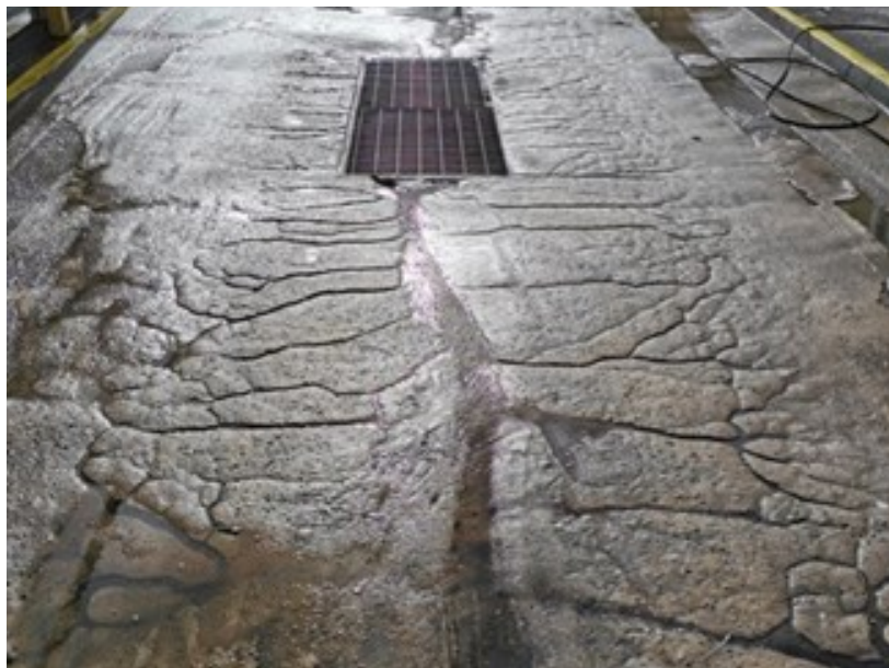
Figure 10: Purpose made water drainage by the petrol station. Surface requires upkeep. Norfolk
