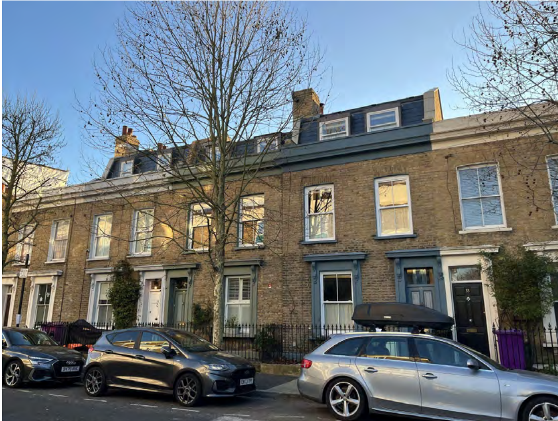
Examples of roof extensions within a Tower Hamlets conservation area that match traditional designs
